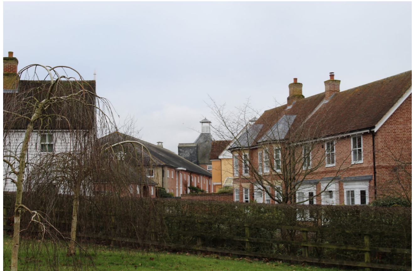
Figure 74 Listed maltings buildings at centre of development
