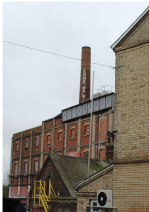
Figure 119 EDME Chimney from Mistley High Street along with maltings building South east of EDME
