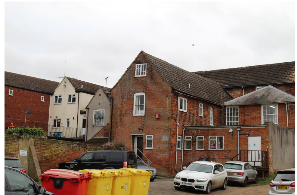
Figure 145 Parking for residents and businesses, North Street
