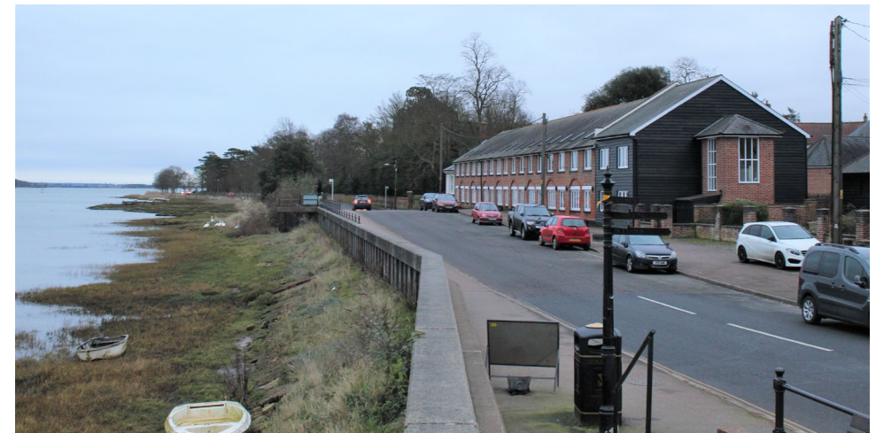
Figure 82 View along the Walls from Manningtree into Mistley
