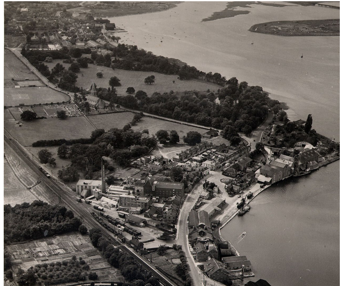
Figure 16 Aerial shot of Mistley with Manningtree in distance. Many of the maltings buildings of both Mistley and Manningtree are visible along the riverside. This photo shows the green gap between the two settlements (EROX172-19 IMb244-1-17).
