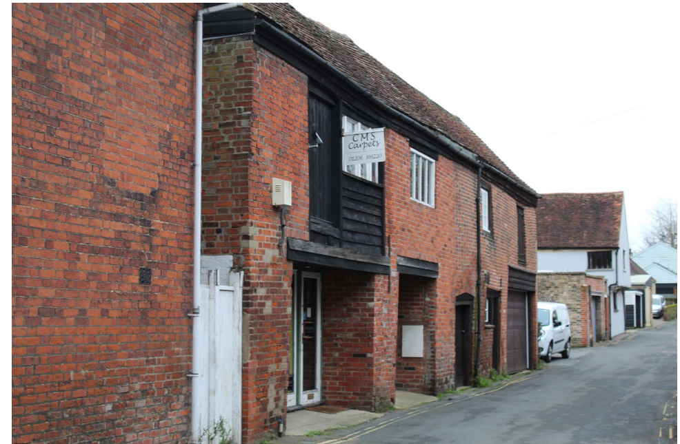
Figure 49 Industrial buildings on Stour Street featuring repaired brickwork and black weatherboard infill
