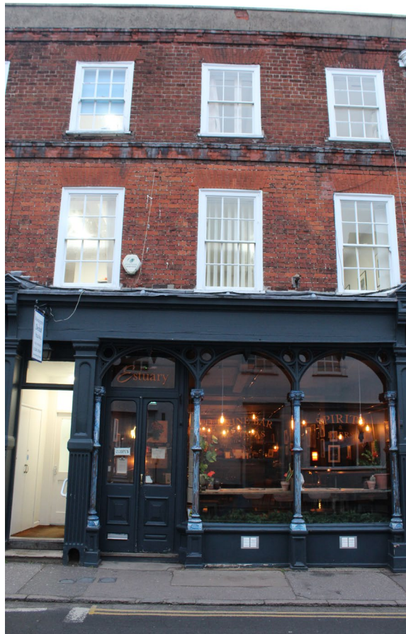
Figure 147 Historic shop frontage, Manningtree
