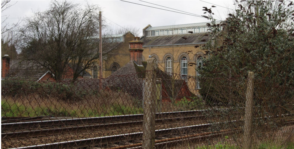
Figure 69 Pump House and railway, Lawford Water Works
