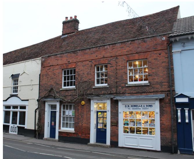
Figure 148 Historic shop frontage, Manningtree
