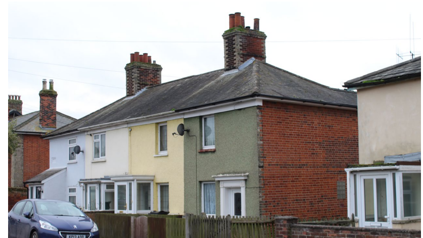
Figure 128 Examples of natural slate roofs within this Character Area
