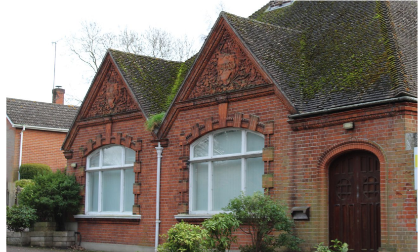
Figure 71 The Bungalow, Lawford Water Works
