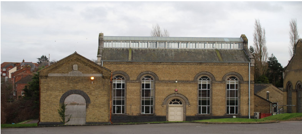
Figure 70 Pump House, Lawford Water Works
