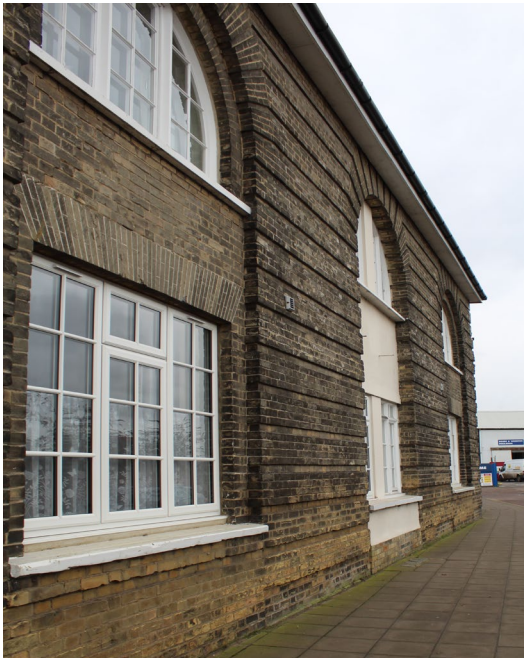
Figure 33 Grade II listed former warehouse to the east of south street
