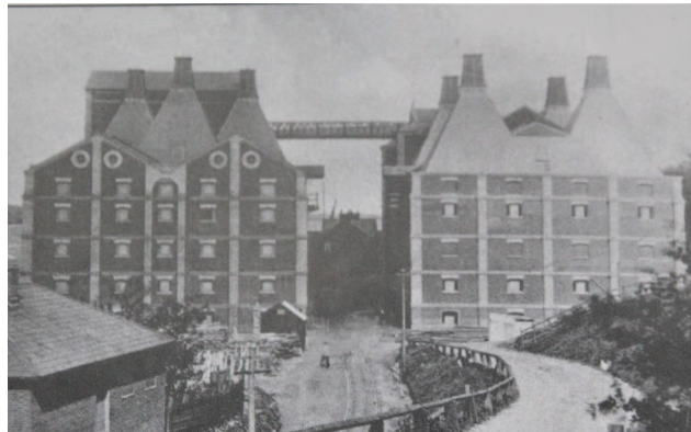
Figure 11 Maltings to the east of the quayside, Mistley
