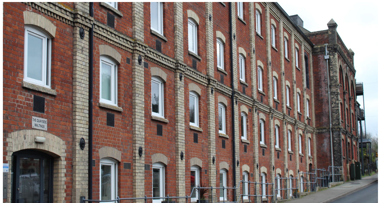
Figure 115 Southern face of Maltings and Kiln 1 (The Quayside Maltings) fronting the High Street
