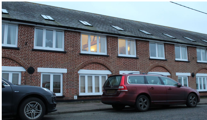
Figure 76 1-10 Brooks Malting with partially infilled arches
