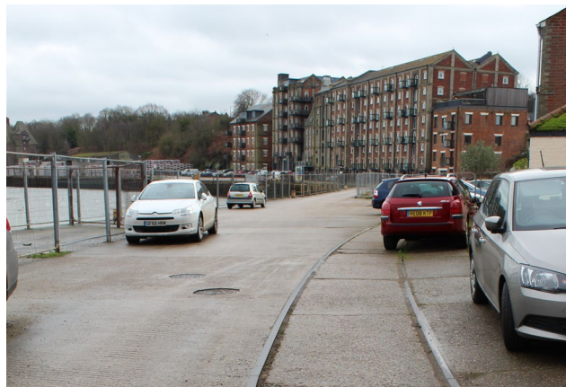
Figure 110 Surviving rails of the tramway which once spanned the quayside at Mistley
