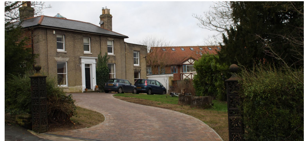
Figure 59 Gault brick frontage of Number 23 Colchester Road at the entrance of the former Lawford Iron Works
