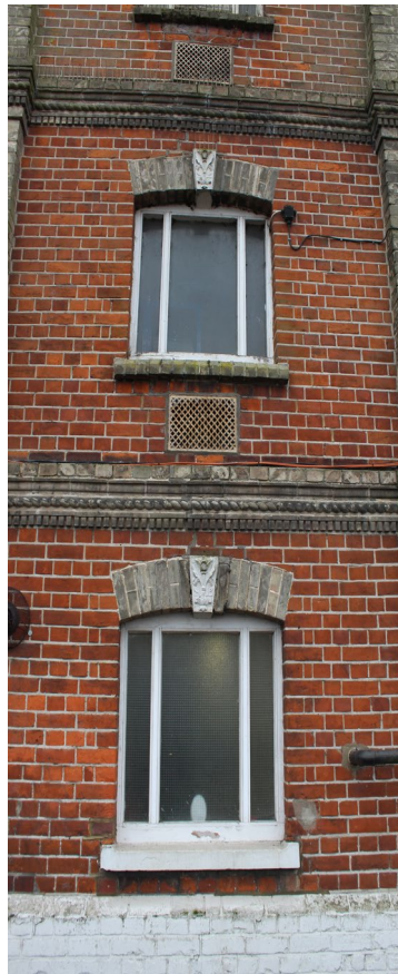
Figure 112 Red brick elevations with yellow stock brick details
