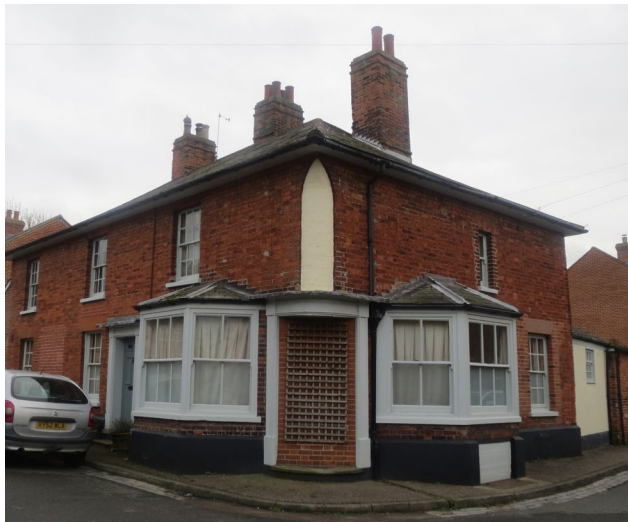
Figure 126 Former Lord Denman Inn, California Road
