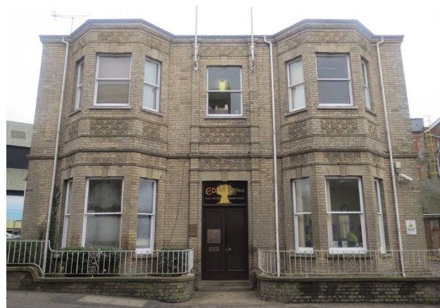
Figure 117 EDME House with decorative bricks and large bay windows
