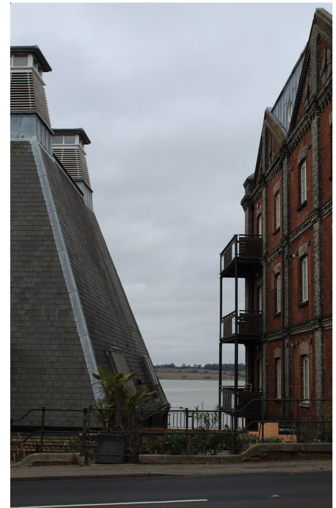
Figure 111 Nineteenth century converted maltings buildings with River Stour behind
