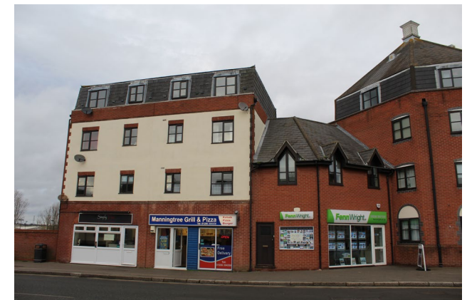
Figure 58 Blue brick window heads and sills
