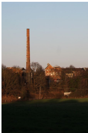
Figure 120 EDME Chimney from Green Lane
